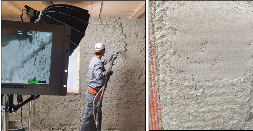
Fig. 3. Application of reference render akurit TRI-O-Therm L [7]
